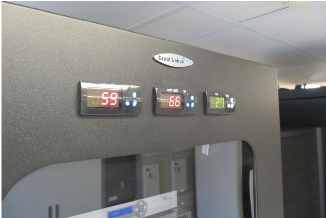
The CLWCE has easy to read enclosure diagnostic indicators.
